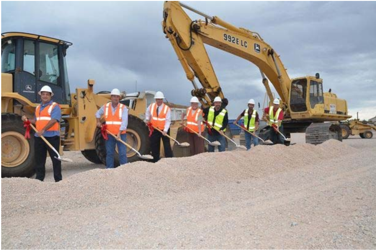
CCSD Board of School Trustees Clerk Carolyn Edwards, along with Associate Superintendent of Facilities Blake Cumbers and representatives from Martin-Harris Construction, breaks ground on a new elementary school near Dean Martin Drive and I-15.
