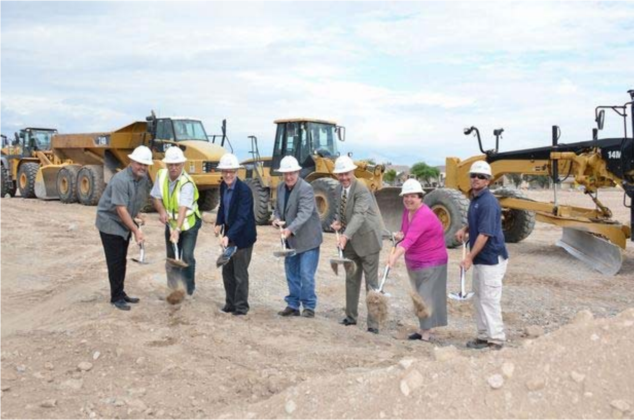
CCSD Board of School Trustees President Deanna L. Wright, along with Associate Superintendent of Facilities Blake Cumbers and representatives from APCO Construction, breaks ground on a new elementary school near Spencer Street and Pyle Avenue.
